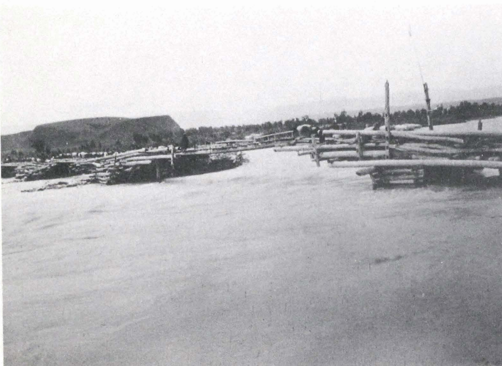
A precarious crossing on the Tekes river.
